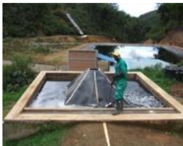
Reactor UASB
